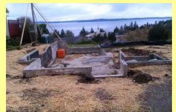
KHM Construction—W Seattle project—what a view the new house will have!
